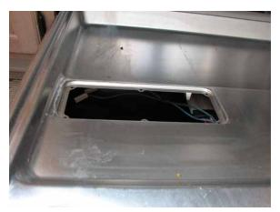
I spent a few minutes cleaning the edge of the hole so that the new unit's rubber seal would be able to do its job effectively.
