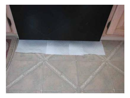
The final step is to make sure nothing leaks!!! As I do with any work that involves water, I use the "dry paper towel" test... Just put a few dry paper towels around the area in question (in our case, the front of the dishwasher), run it through a cycle and make sure that the towels are dry at the end of it all...
